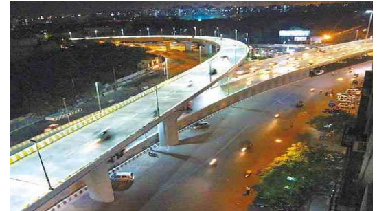
Varacha Road fly over
